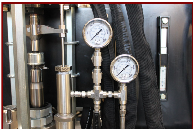
STAINLESS STEEL CATALYST PUMP WITH OVER AND UNDER PRESSURE CONTROLS
